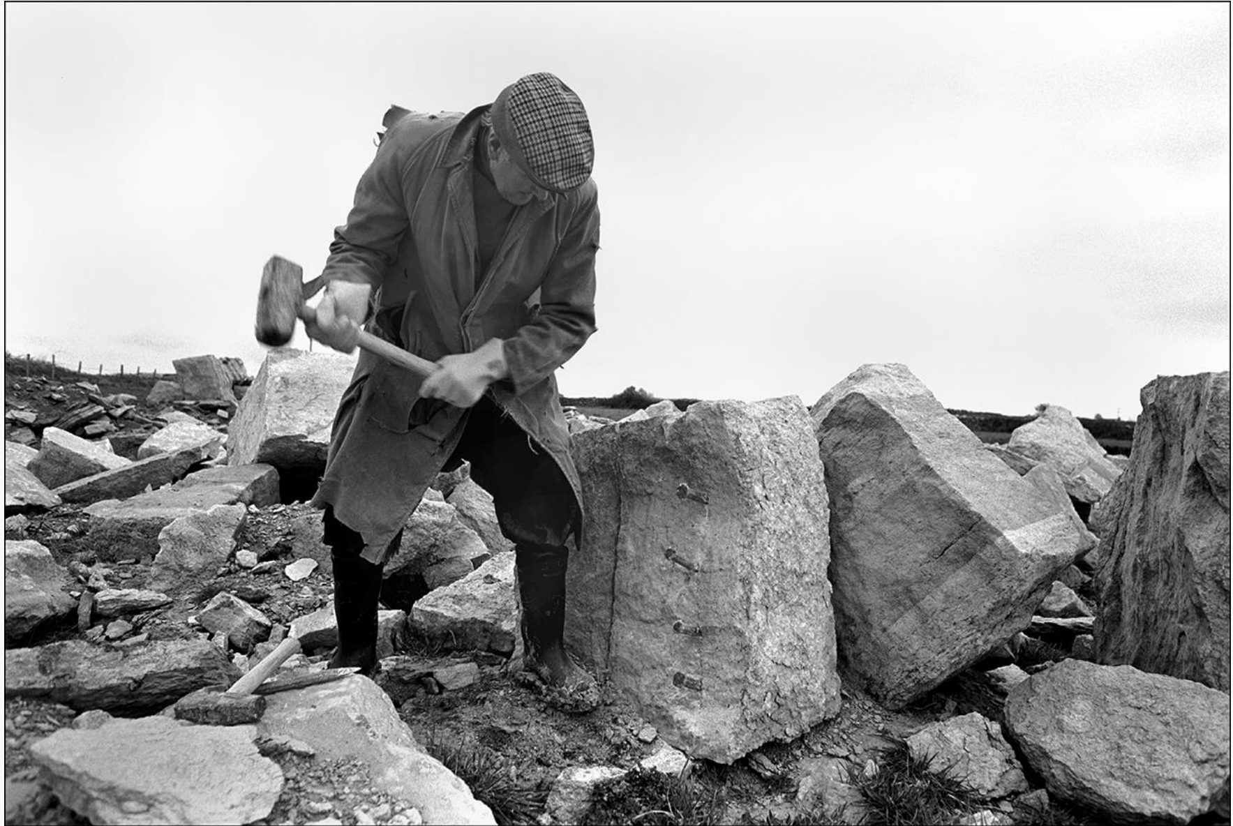
Eric Bower splitting stone with wedges. 1983
