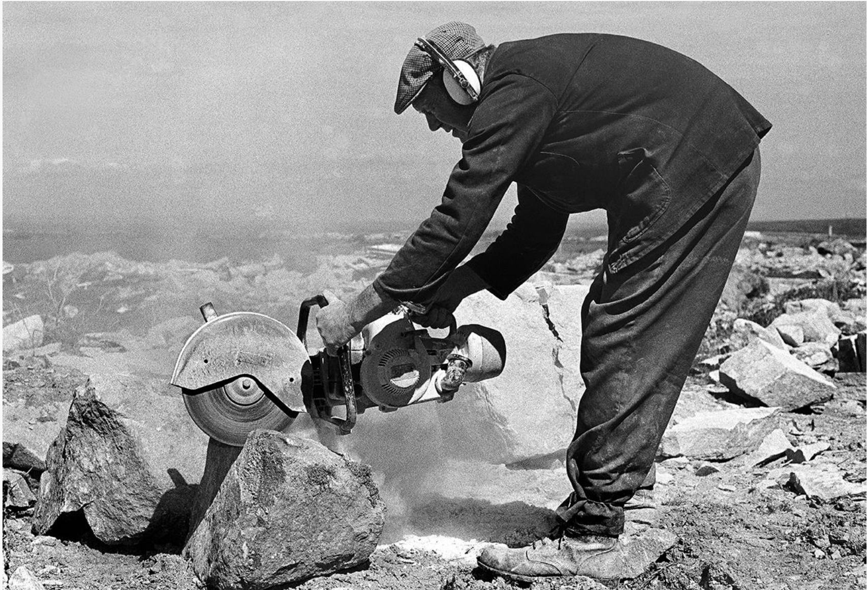
Ron Bower with angle grinder to create a groove for the wedges. 1983
