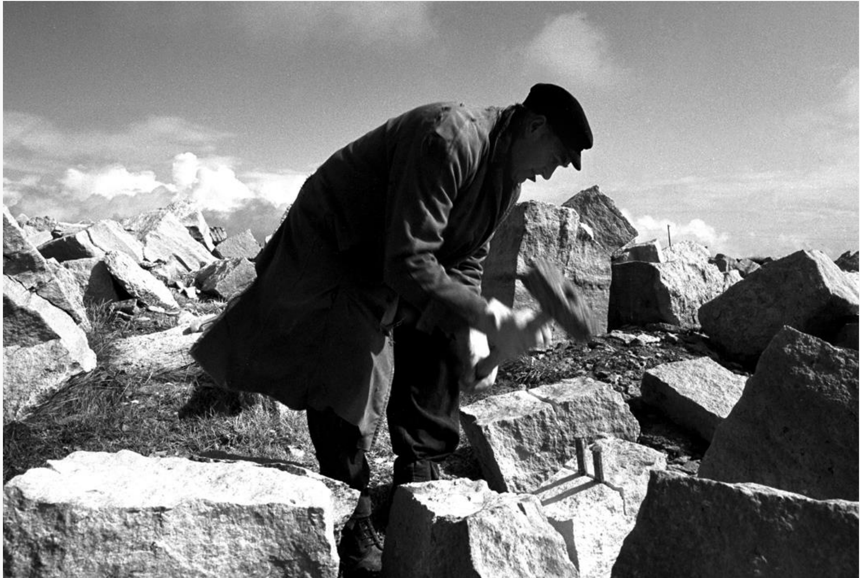
Eric Bower splitting stone with wedges. 1983
