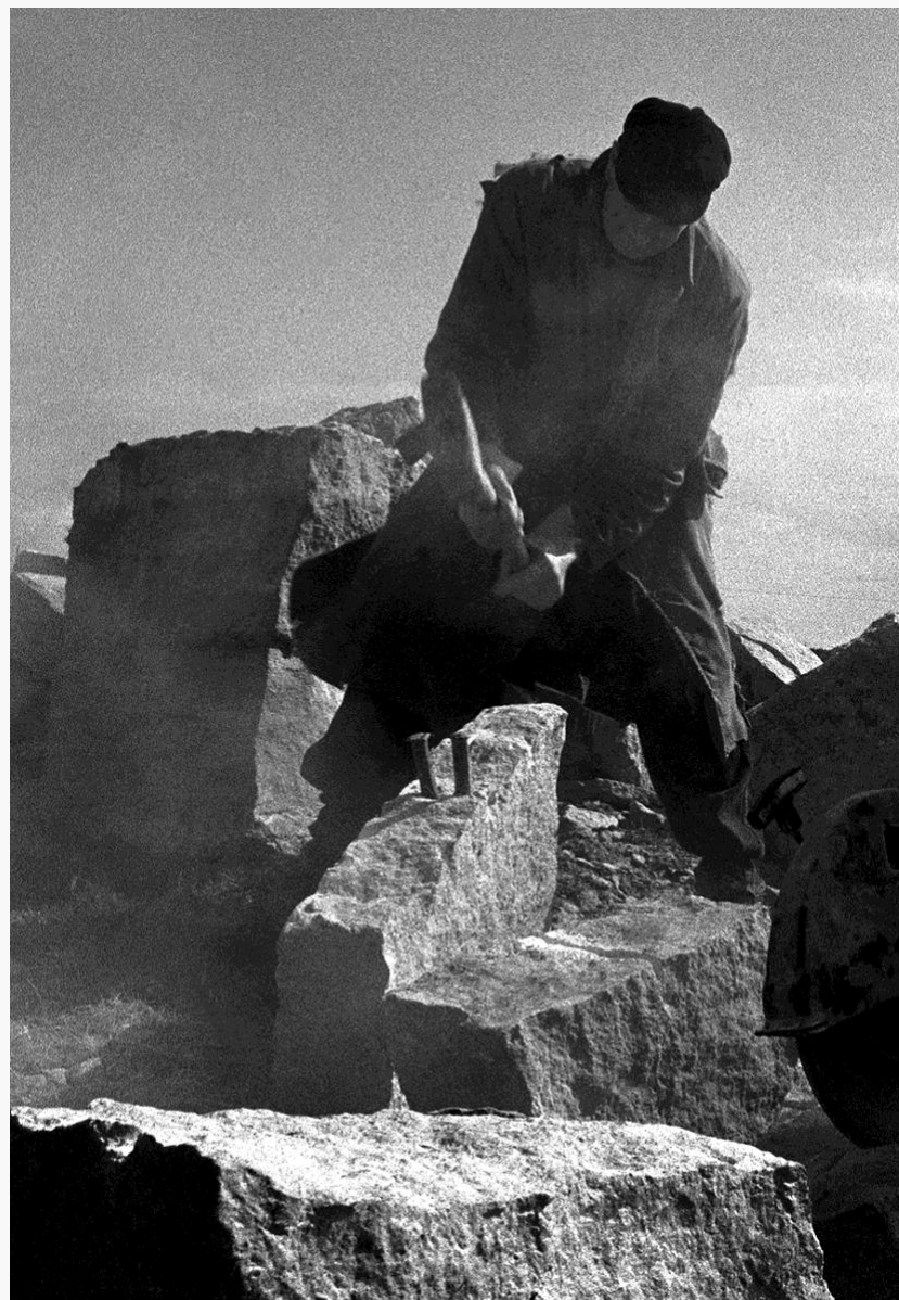
Eric Bower splitting Purbeck stone with wedges, 1983
